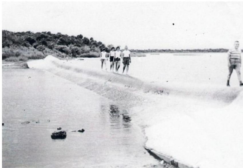
Figure 14. Historic photograph showing tourists crossing the Upper Myakka Dam (8S02273) along the Upper Myakka Lake at Myakka River State Park, after concrete was added to earthen levee. 61
