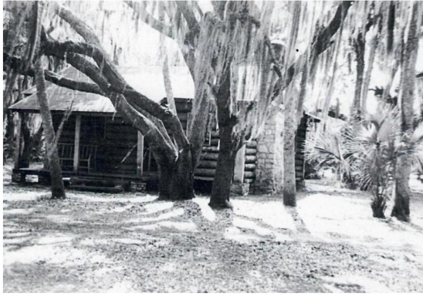
Figure 17. Historic photograph showing cabin constructed by the CCC at Myakka River State Park. 64
